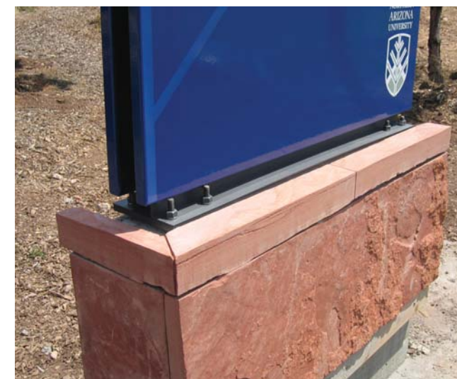
Vehicular Building ID Porcelain panel, metal bracket, sandstone base mock-up
